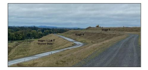
Figure11. 2: Embankments side profile
